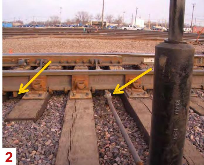
**1: It may be necessary to chip away compacted snow and ice off the tie plate to get the switch to latch and get a switch point that does not gap.**
