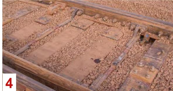
1: Movable point under rail is “cribbed” out and free from obstructions.
