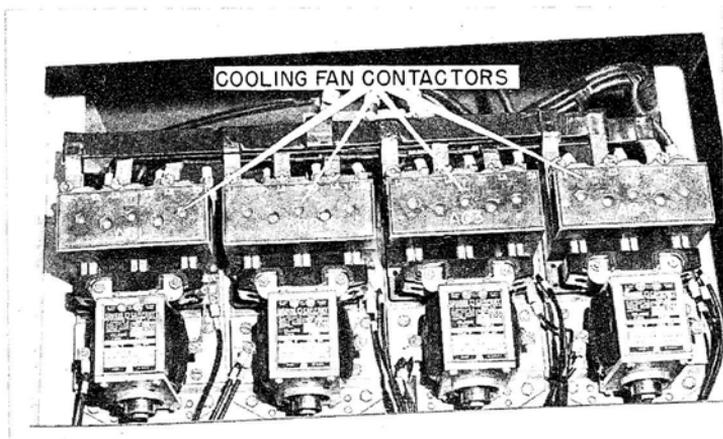
AC Contactors - Water Temperature Controls
